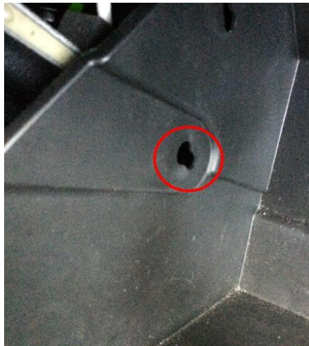
Retaining cylinder removed
