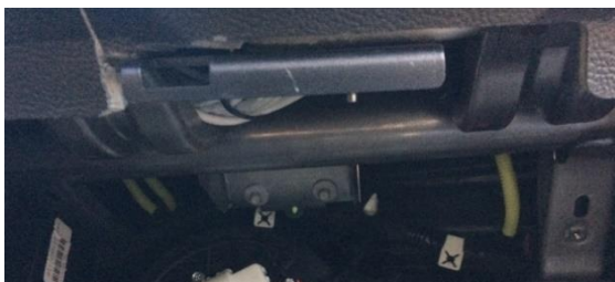
New latch installation
